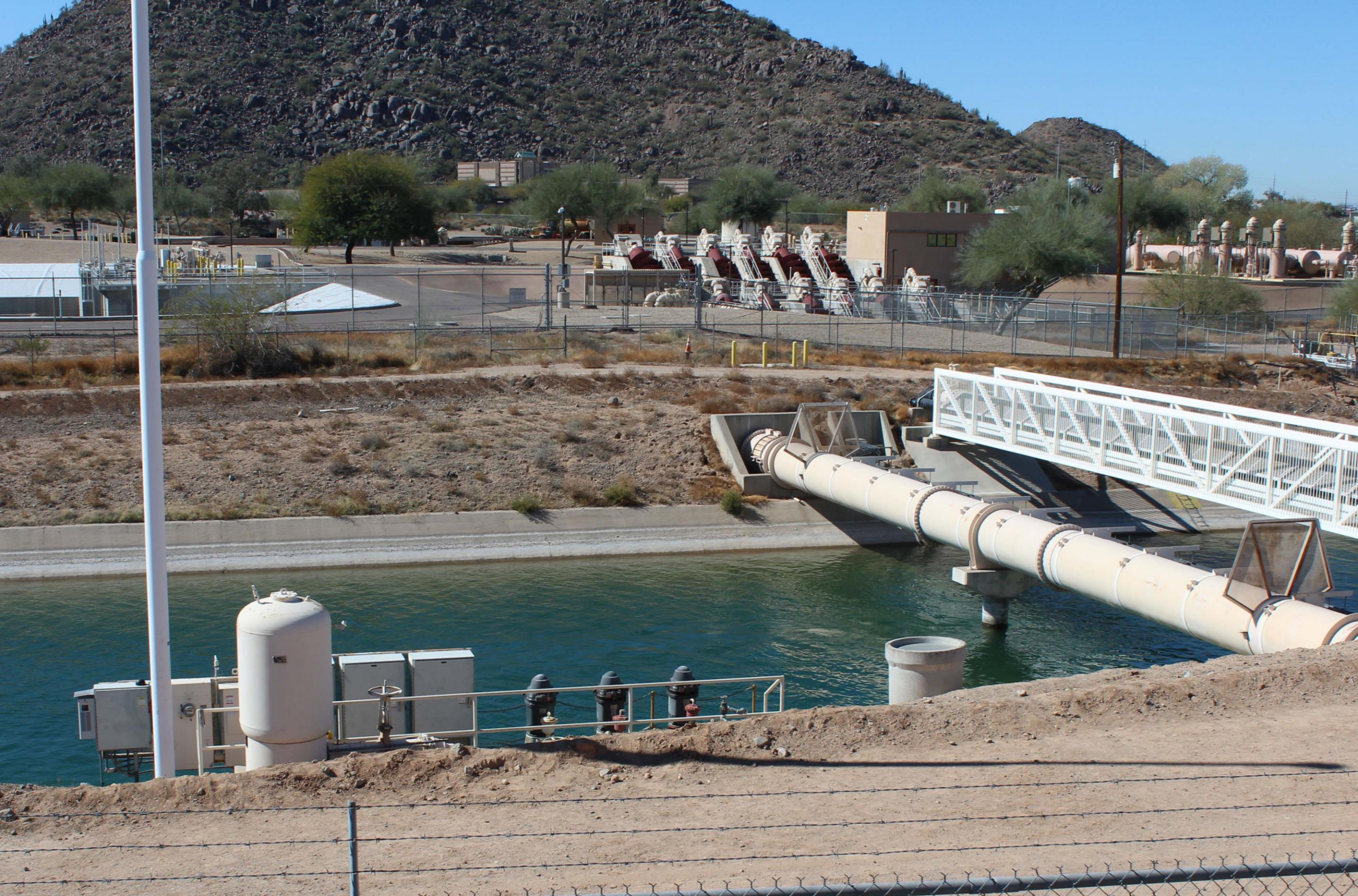
Cave Creek receives its water from the CAP canal at Deer Valley Road. It's pumped uphill 600 feet and 12 miles to the Town of Cave Creek.
