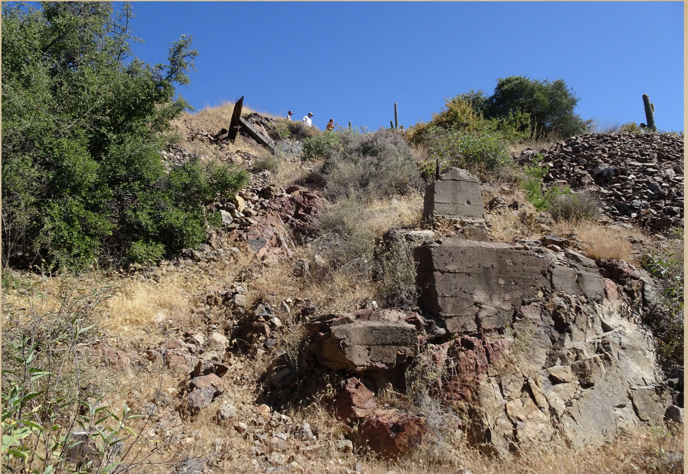
Broken concrete footings, timbers and cables can still be seen on the bank below the trail. The title slide in this tour is a view of the mine and tailings from the creek bed below.
