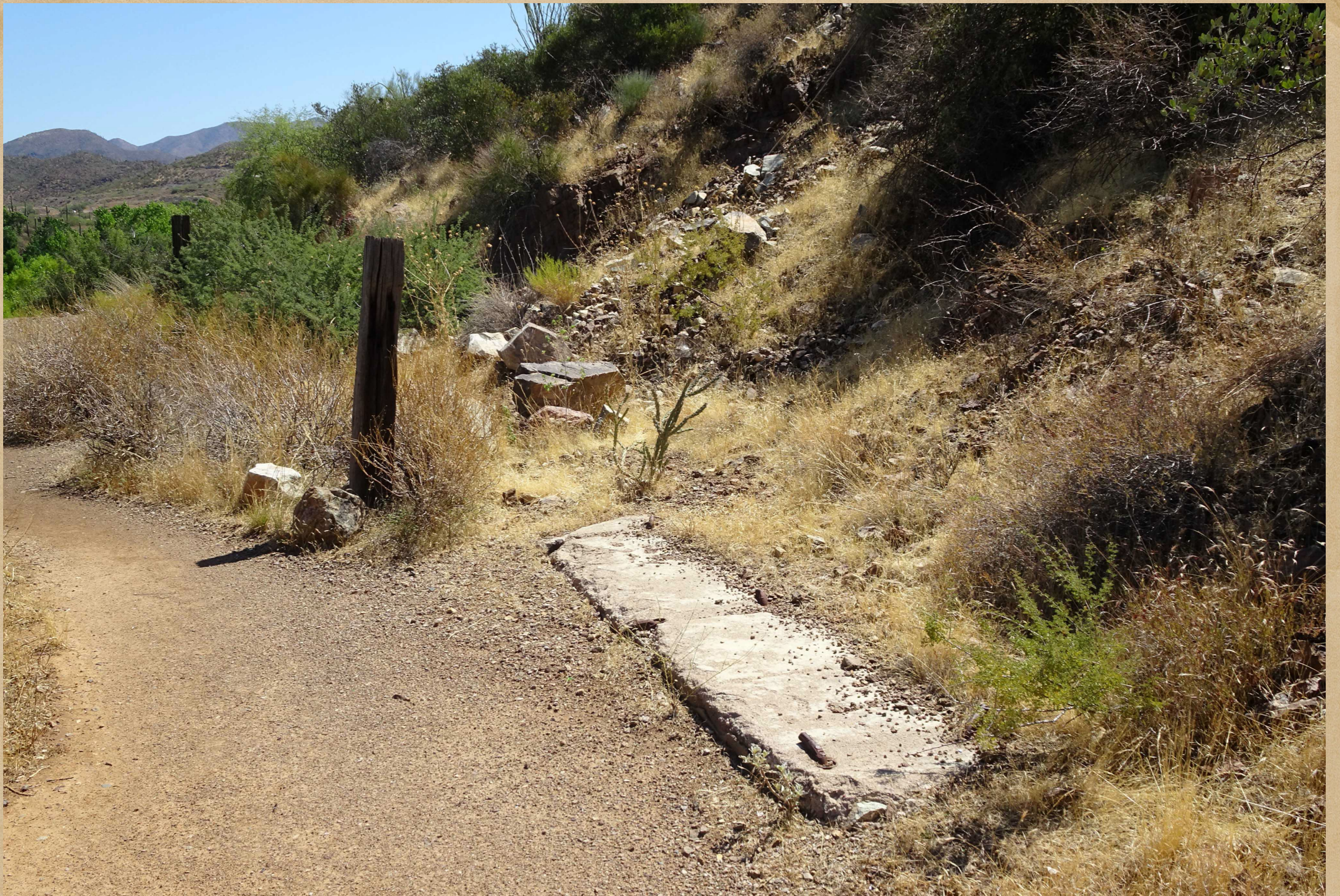
Weathered wood posts and the concrete foundation were a part of the Maricopa Mine structure.
